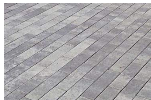
C GRAY UNIT PAVERS TO MATCH R.O.W. IMPROVEMENTS DESCRIPTION: PERMEABLE UNIT PAVERS COLOR: GRAY SUPPLIER: BORGERT SIZE: 5' x 10'
